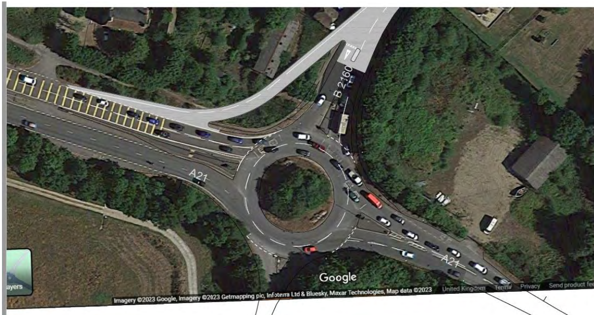
Figure 8-3 – Kippings Cross Left Turn Slip Lane
